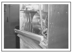
10. Remove the 2 sheet metal screws that attached the blower to the bottom of the blower shelf. (1/4" Socket)
