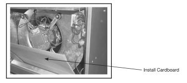
6. Remove the 3 sheet metal screws which attached the blower to the blower shelf located in the air handler control box. (3/8" Socket).
