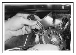
12. Remove the motor assembly from the air handler.
