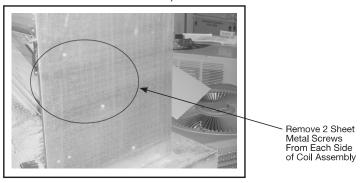
9. Tilt the coil assembly forward. (NOTE: Depending upon the amount of slack in the refrigerant lines, the system may have to be evacuated and the suction and liquid line of the air handler may have to be uninstalled from the system in order to prevent damage to the refrigerant lines which could result in a total loss of refrigerant)
