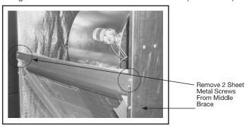
8. Remove 4 sheet metal screws (2 on each side of the air handler)
